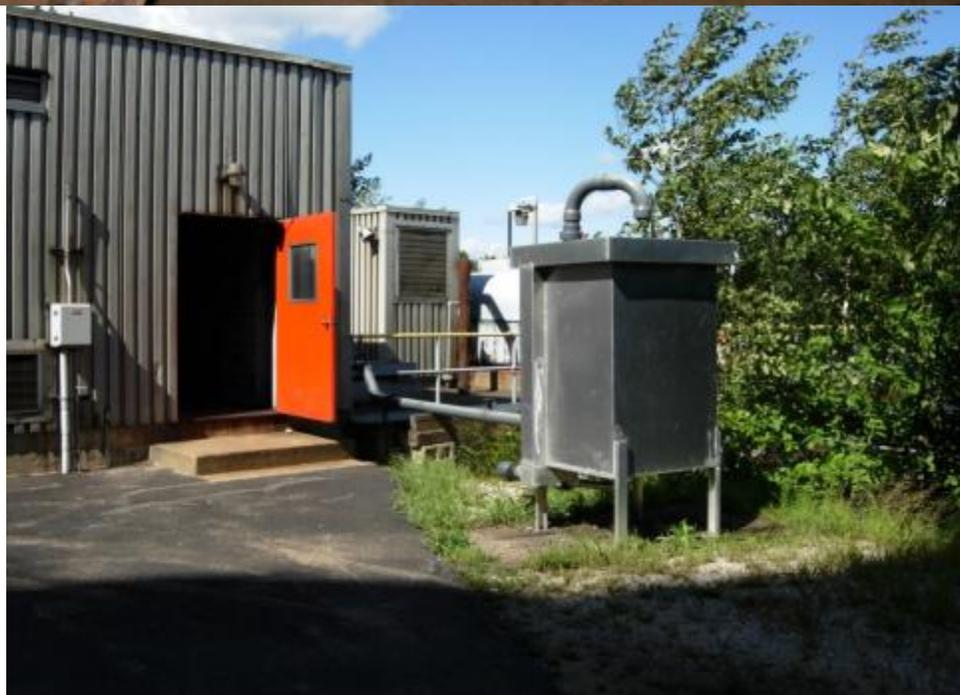
Figure 2-5. Location of the tap (top panel) supplying condenser flow into the entrainment sampling tank (bottom panel) from the main condenser supply lines within the CWIS control sampling location at Merrimack Station Unit 1.
